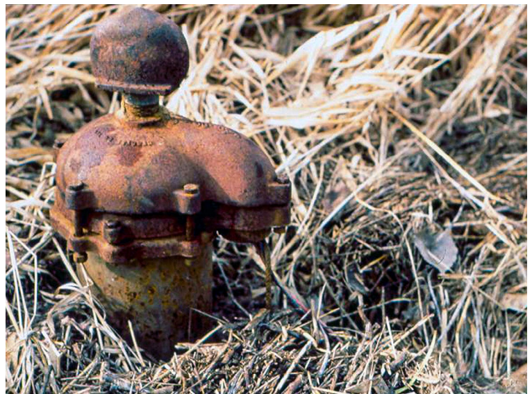
Figure 2. A vented well cap over the casing protects the water supply from surface water and other contaminants.
